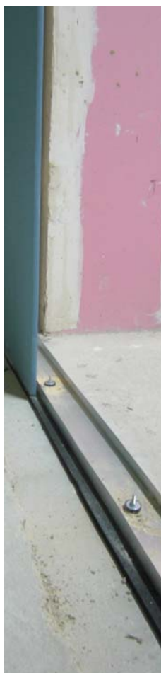
Above: FAVIM used as full area isolation of a floor.
