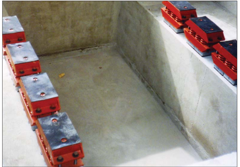
Precision Roll Grinding Machine on FSL Coil Spring Isolator with FV Damper Isolated Foundation System.
