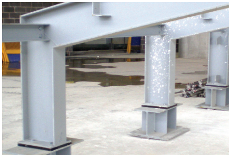
Above; acoustic bearings and washers for cinema raked seating. Right; Acoustic bearings pads for a 7 storey office and residential building.
