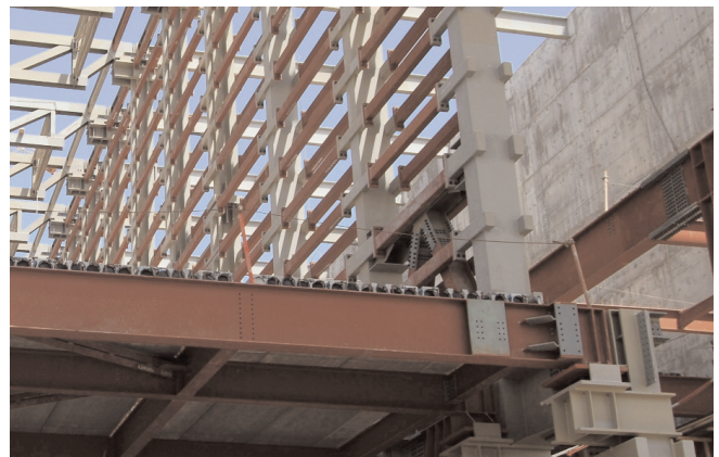
Low frequency acoustic & slide bearings for floor & roof structure of QECC project.
