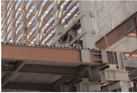
Low frequency acoustic & slide bearings for floor & roof structure of QECCC project.
