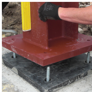
Above; acoustic bearings and washers for cinema raked seating. Right; Acoustic bearings pads for a 7 storey office and residential building.
