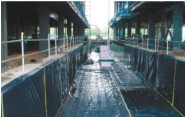
ISOMAT isolated foundation for large Cerutti printing press
