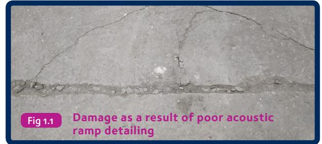
**Fig 1.1** Damage as a result of poor acoustic ramp detailing
